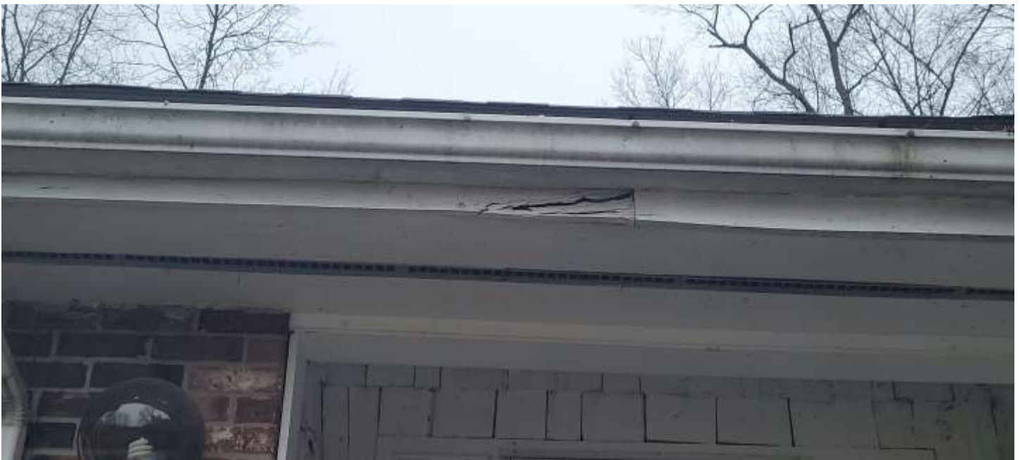
Soffits here are showing wear.
