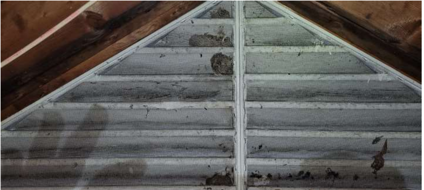
Attic vent has a screen. Also some dead hornets nest on the other side of the screen.
