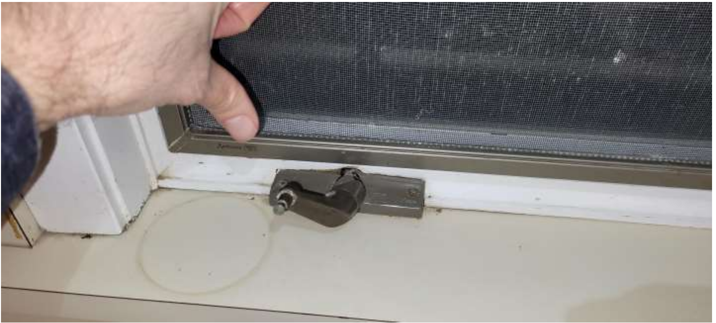
This window opener is broken.
