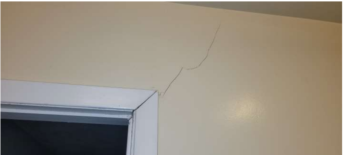
Crack in the wall between the master bedroom and master bathroom. I don't think this is a structural issue. There was also no translation of this crack to motion of the foundation directly underneath this in the foundation area.
