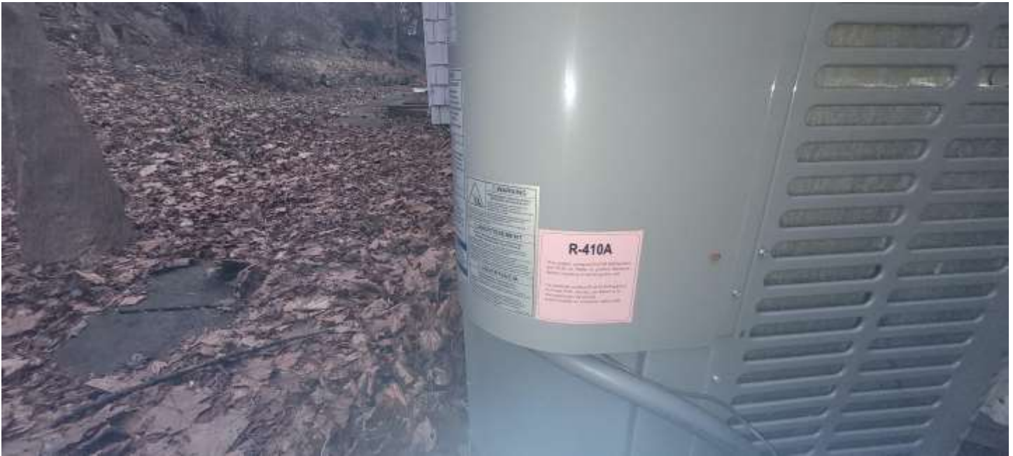
Condenser datacard. R-410A refrigerant.
