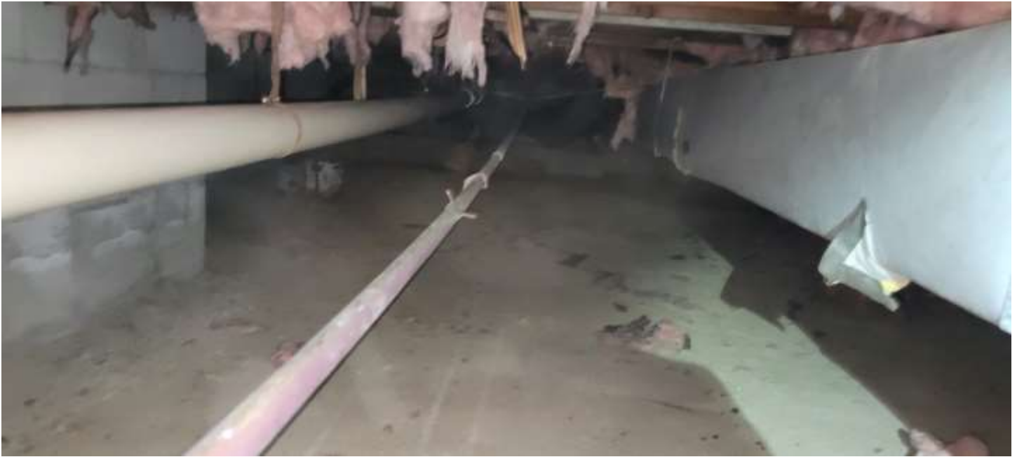
Looking toward the garage wall. That water line should be supported better.
