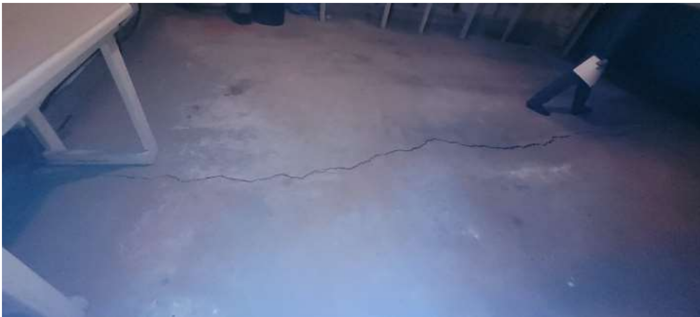
Garage slab had two large cracks.
