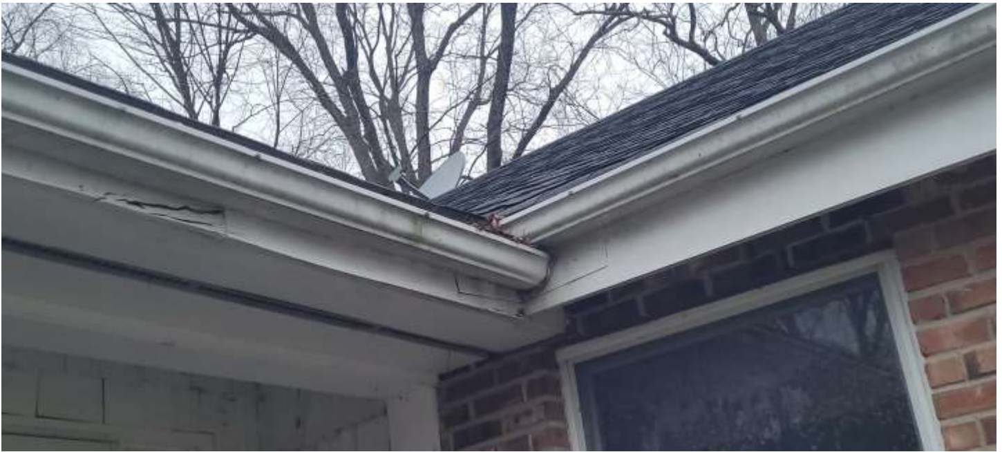
Soffits here are showing wear. Gutters are clogged.
