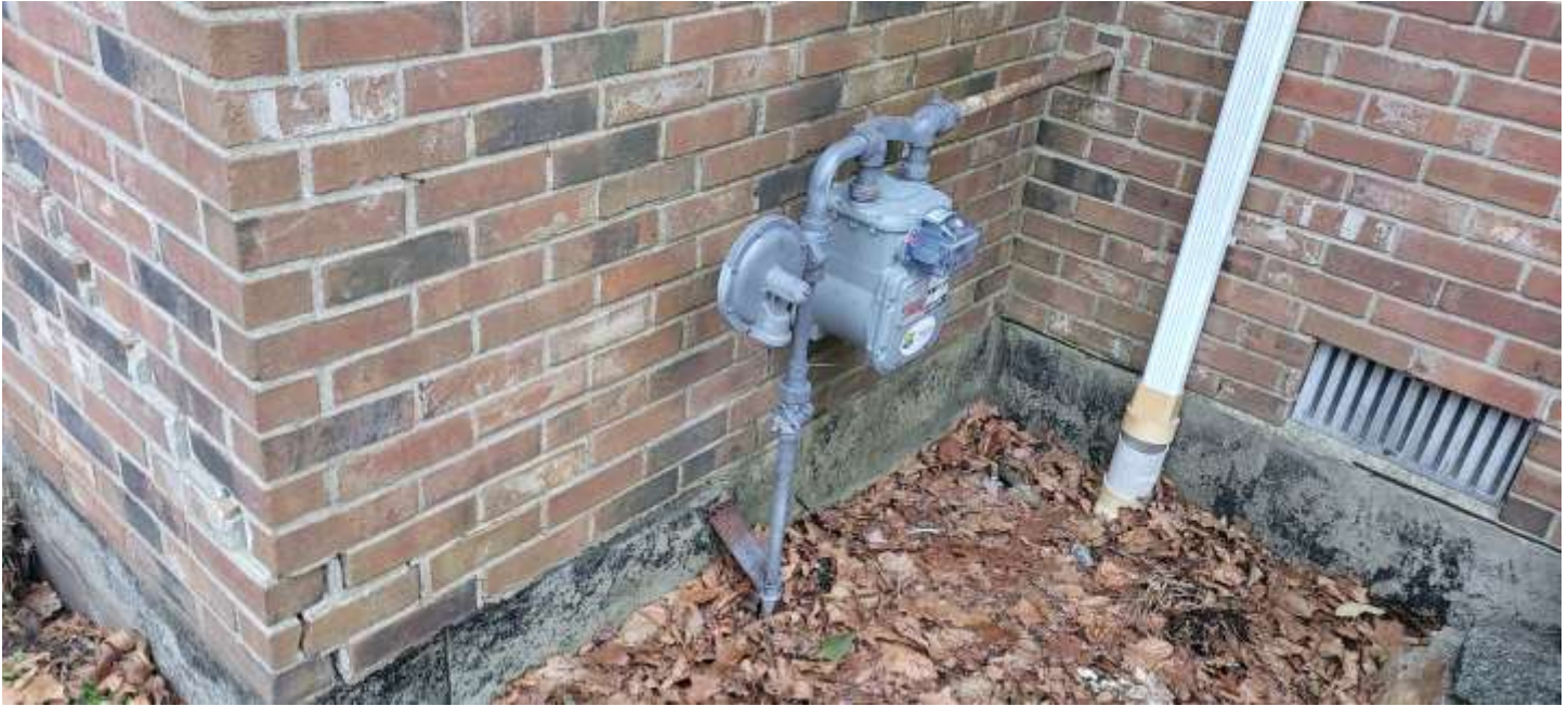
Gas meter and shut off. Notice the cracking of the bricks of the garage.
