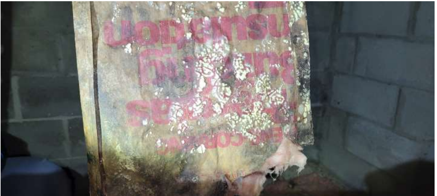
There is some mold in this basement. This is consistent with a very humid basement, and the presence of water.
