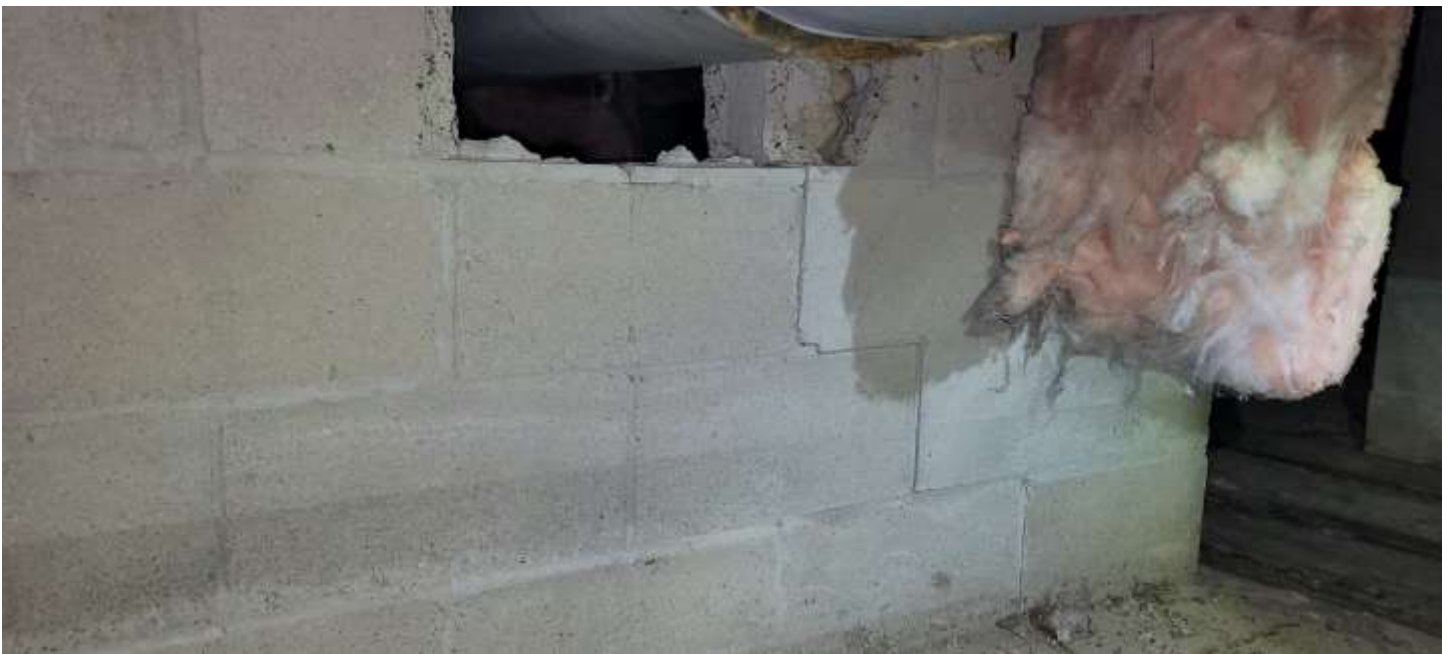
Somewhat larger crack here. This is also reflected in the bedroom above it. This seems to have moved about 1/4"-3/8".
