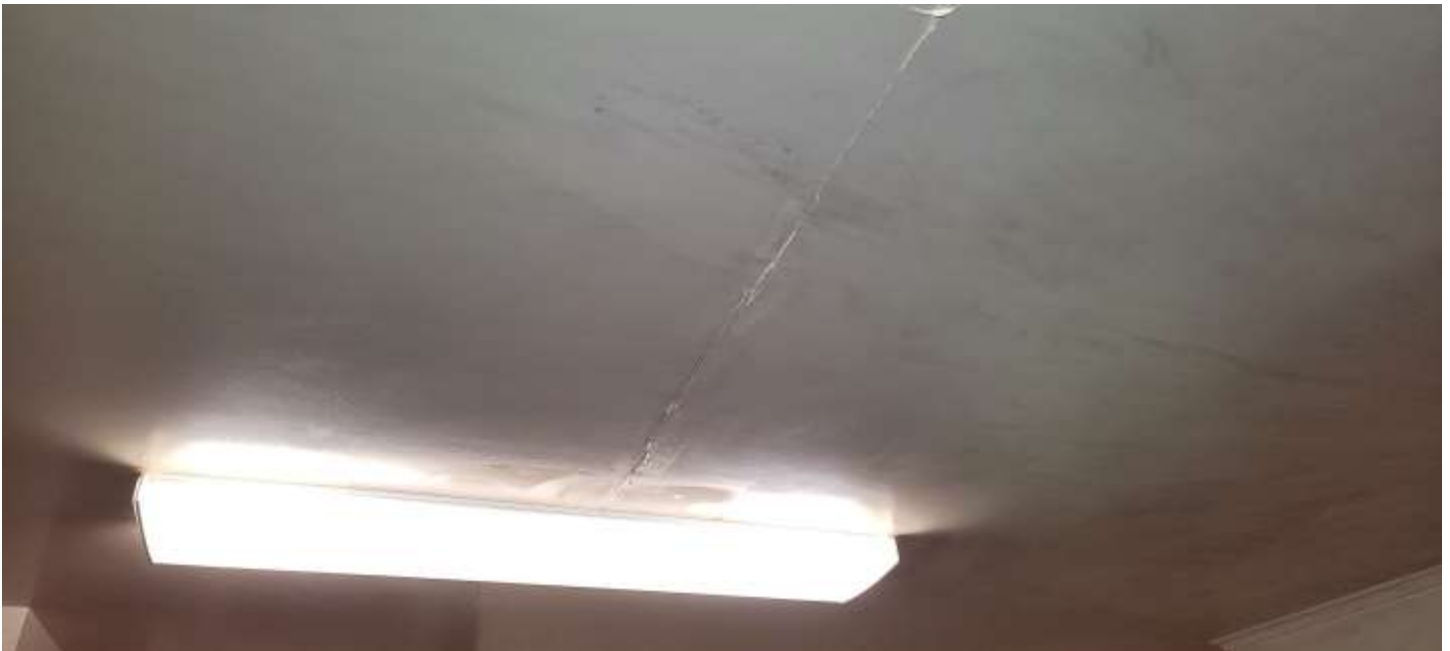
Kitchen ceiling. I don't think that crack is structural.
