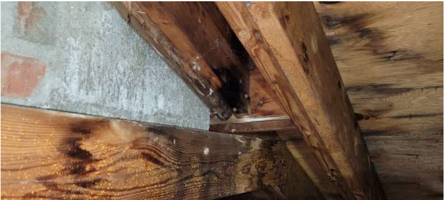
Chimney in good visual condition. Typical. There seems to be one area in the flashing where water got in. Consider re sealing that, if this is a “current” leak.
