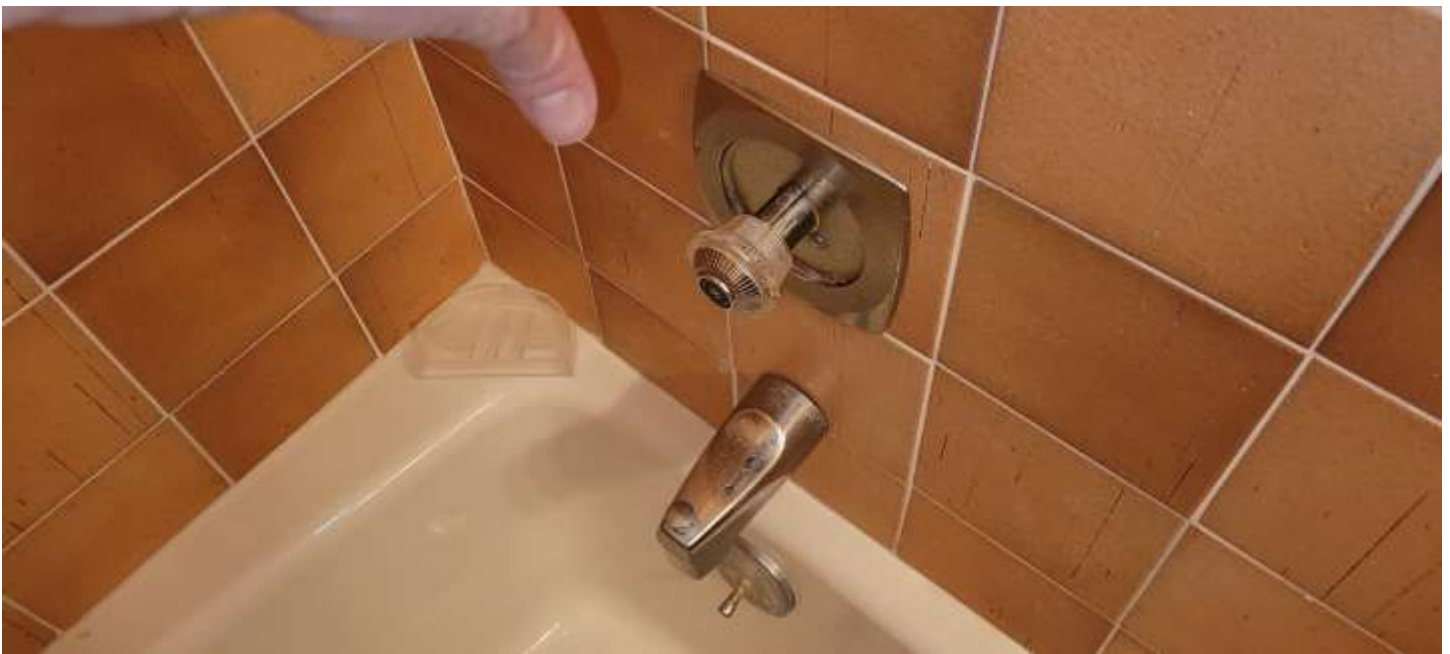
This faucet actuator is sticky, and I could not get it to operate.
