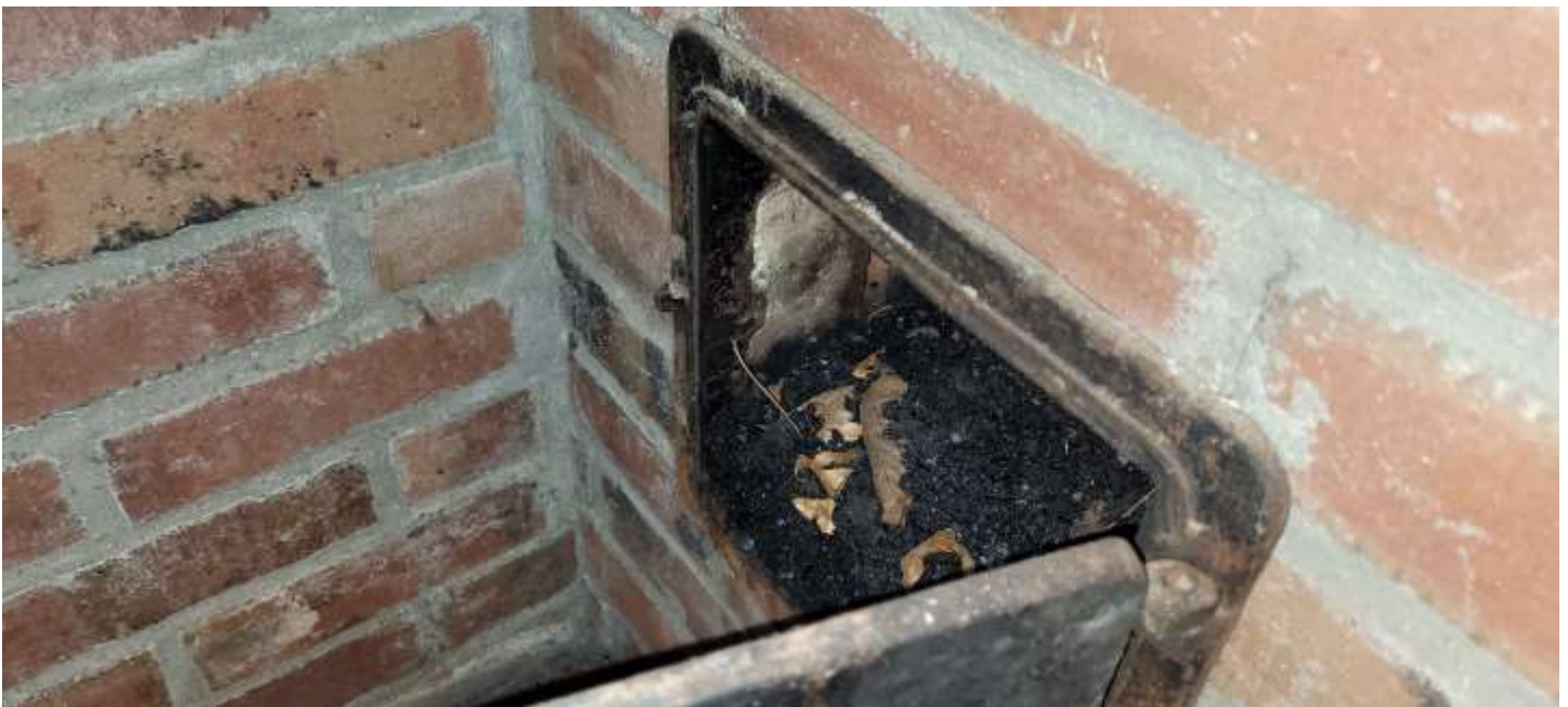
Fireplace clean out needs to be cleaned out.
