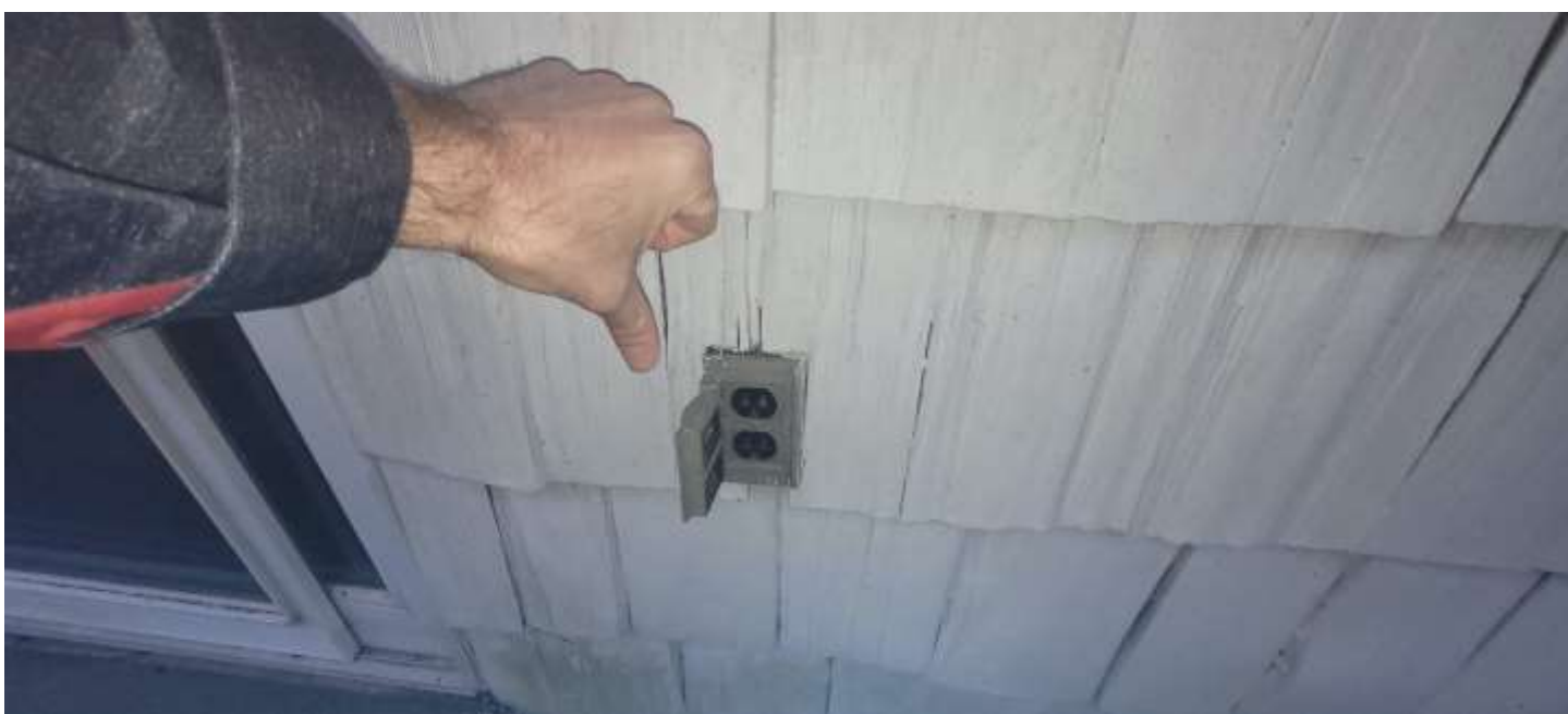
This outlet should be GFCI protected.
