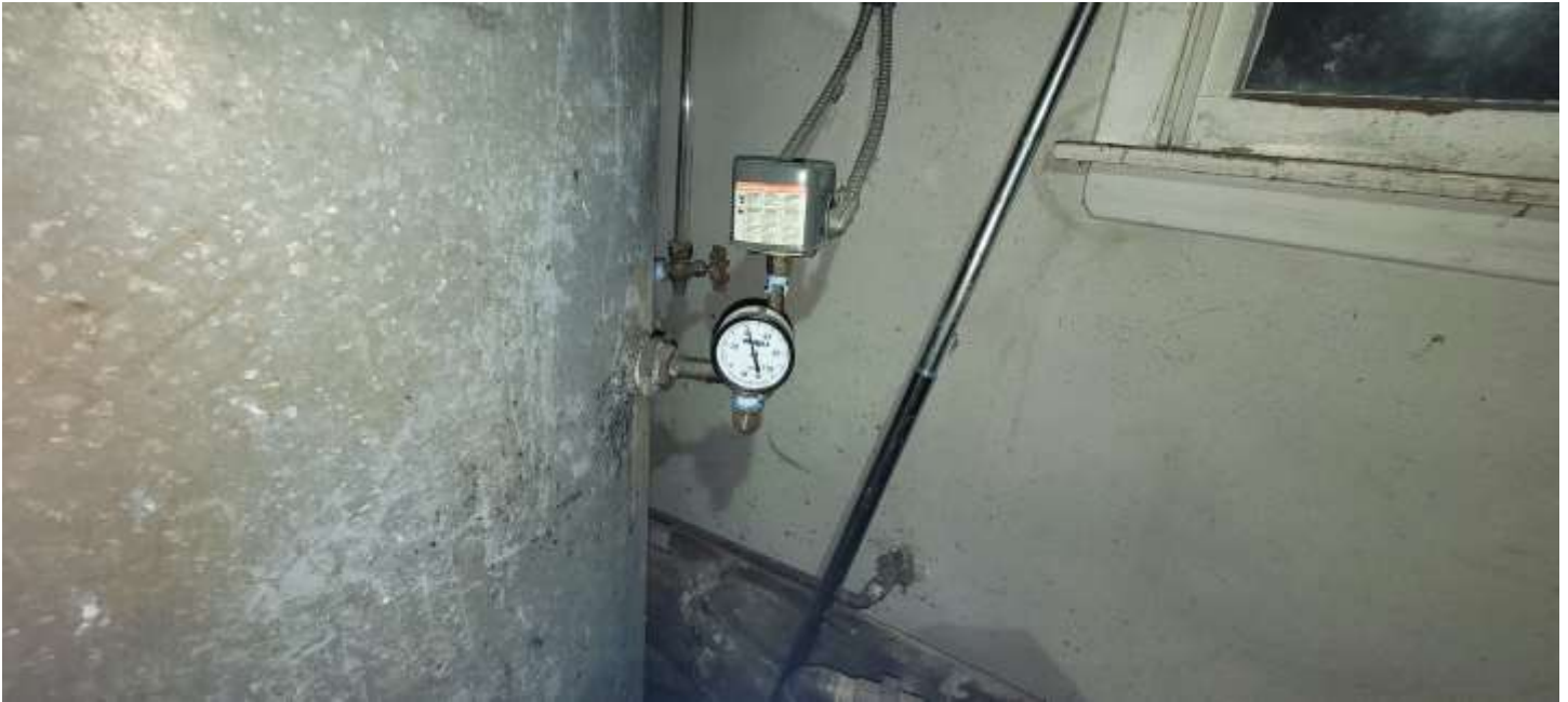
Static water pressure from the systems pressure gauge.
