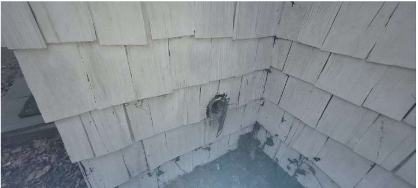
Painted wood generally well maintained and in very good condition. The dryer outlet is clogged.
