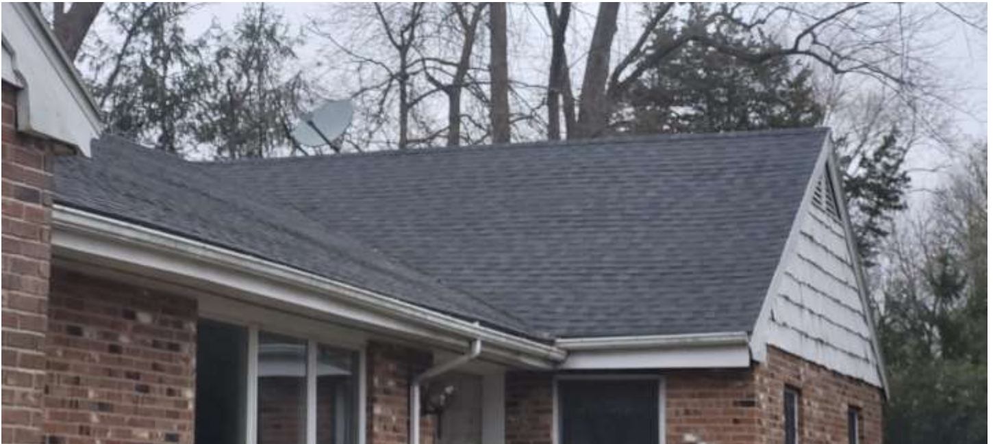
Soffits show some wear here. Gutters are showing signs of being clogged. Shingles in good visual condition. I suggest these gutters be cleaned, and repaired.
