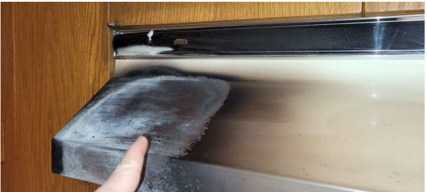
Notice the burns on this hood vent. I suspect this is strongly correlated to the smoke stains on the ceiling about 3 feet away.
