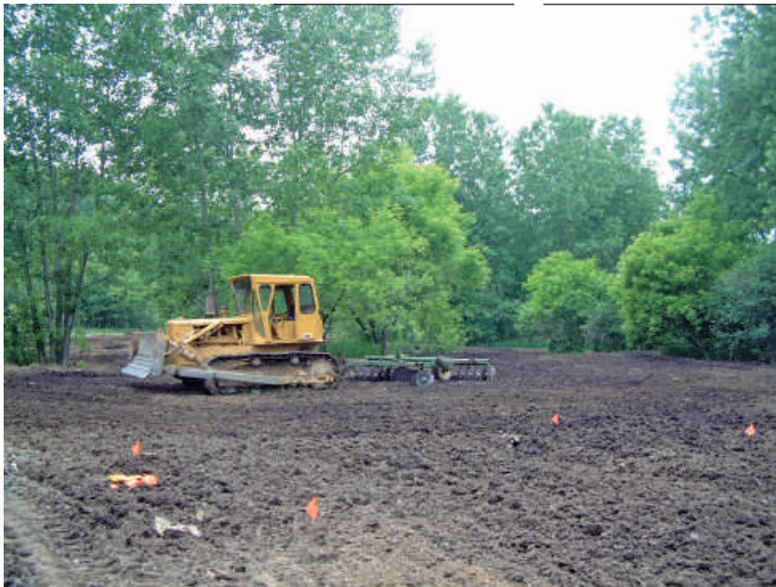
FIGURE 4. Using dozer-drawn harrows on former industrial dump site to prepare for hybrid willow planting.
