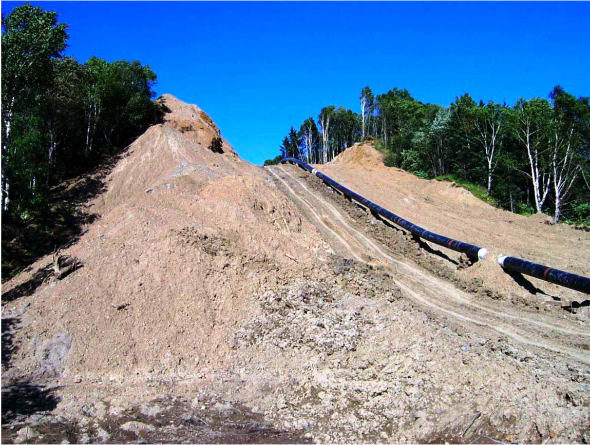
FIGURE 2. An example of a linear-type disturbance: The Sakhalin II oil and gas pipeline and fiber optic right-of-way. Sakhalin Island, Russia.
